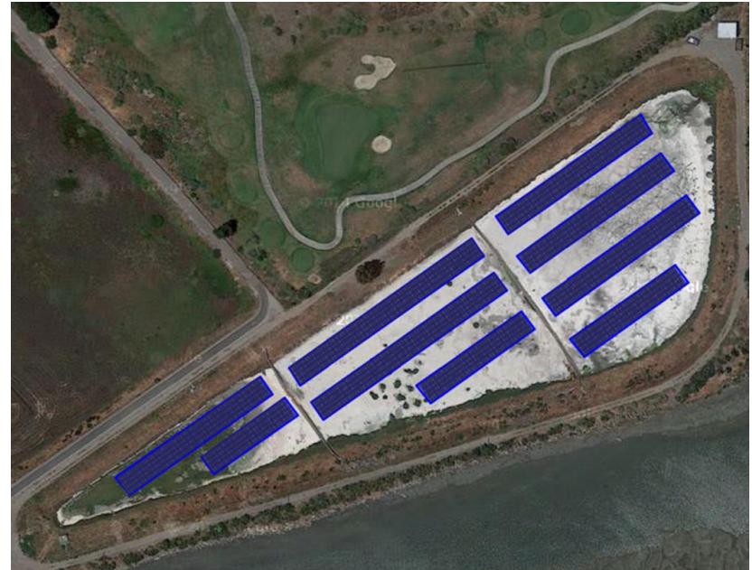
Water Pollution Control Plant
