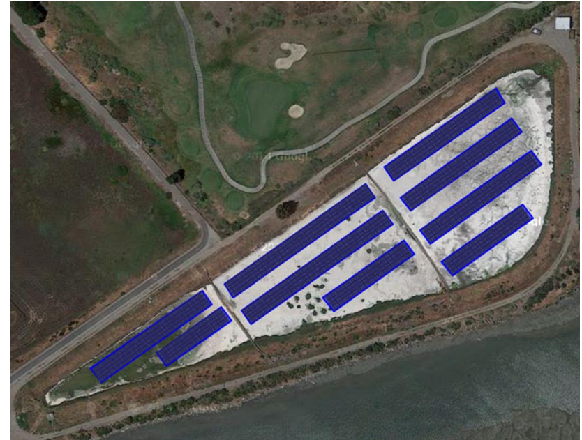
Water Pollution Control Plant
